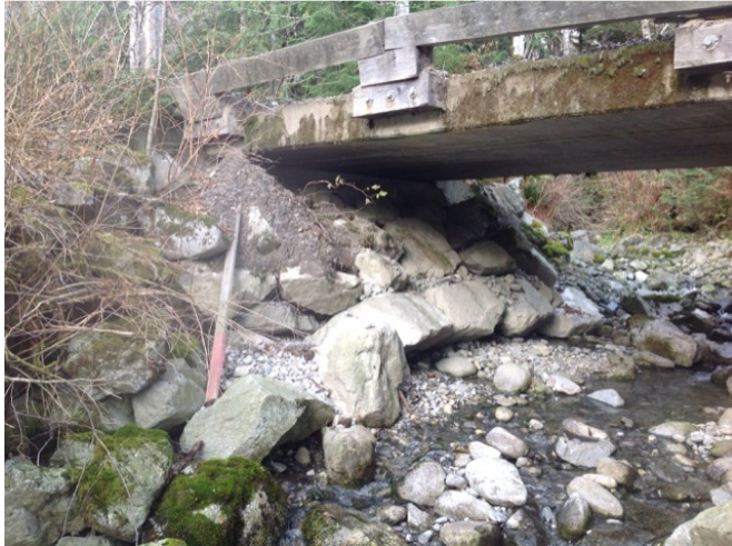
Right Bank Abutment when facing downstream
