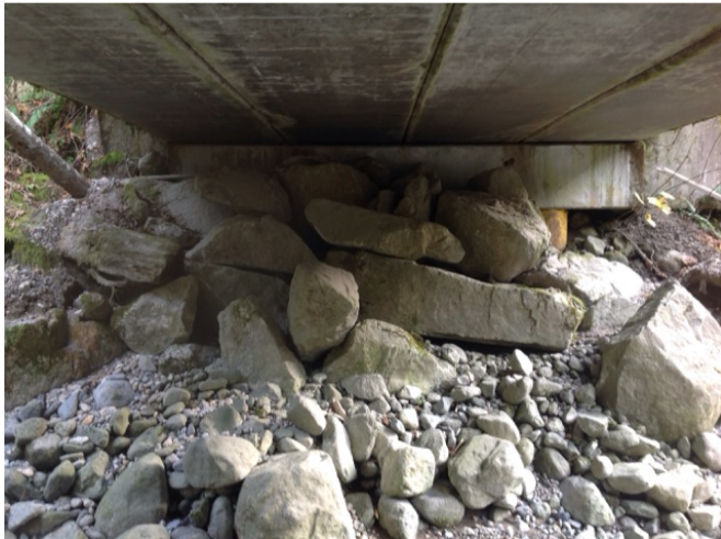
Left Bank Abutment when facing downstream
